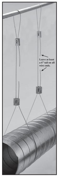
As a matter of sound engineering practice, the Dyna-Tite assembly must be located no closer than 12 inches to the suspension point. In the case of round duct, where the wire rope encircles the duct, the Dyna-Tite must be located the distance of one diameter from the duct wall.
