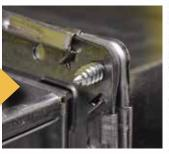
The teardrop shaped cut out of the corner with the proprietary bolt pull the connection together and lock it in place without the use of a nut, using a convenient cordless impact driver.
