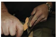
1. Insert the Pittsburgh Lock Opening Tool onto the leading folding edge of the female side of the Pittsburgh seam on a radius fitting and bend the tool back 45 degrees to open the lock for easy insertion of male side of Pittsburgh.
