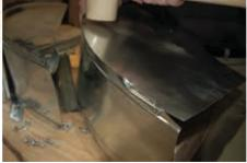
4. Use a wooden mallet or sheetmetal hammer to close the leading edge of the Pittsburgh seam.
